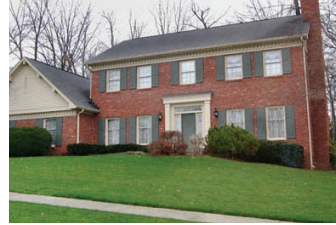
Cut off garage and chimney.
